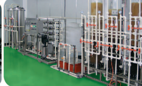
凯泰树脂镜片厂(2m 3 /h镜片清洗用超纯水) Kaitai Resin eyeglass factory (2m 3 /h super pure water equipment for washing)
