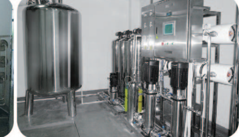
苏州新波生物科技有限公司(2m 3 /h 一级反渗透+二级EDI超纯化水设备) Shuzhou xingbo biological science technology Co.,Ltd (2m 3 /h RO +two stage EDI water purifying system)
