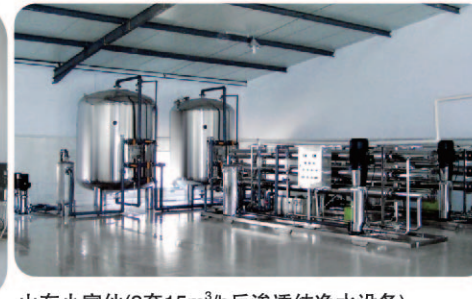
山东小家伙(2套15m 3 /h反渗透纯净水设备) Shandong Sonny(Capacity 15m 3 /h two stage Reverse Osmosis pure water equipment)
