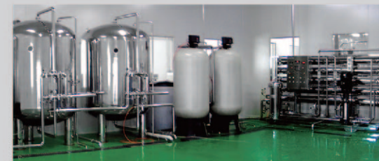
完达山药业(2套15m 3 /h反渗透纯净水设备) Wandashan Medicine (15m 3 /h high pure water RO pure water equipment for medicine factory)
